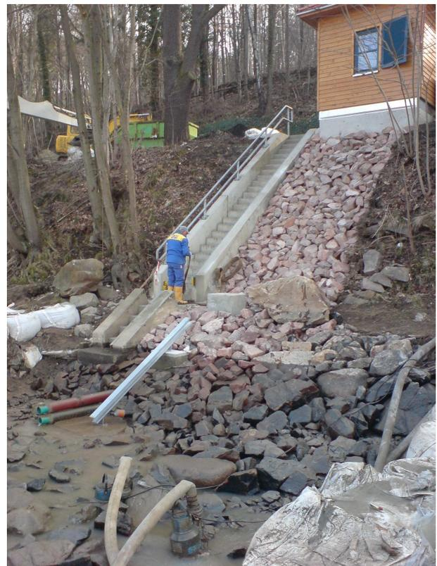
*The gauging station under reconstruction. The carriers for the two SLDs can be clearly seen in the drained channel*
