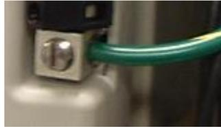
A connection point has been provided for an Earth ground on SL3-1. On SL3-SDI-1 the chassis is the earth ground point. Always connect the earth ground to a suitable ground at the site as described below.
