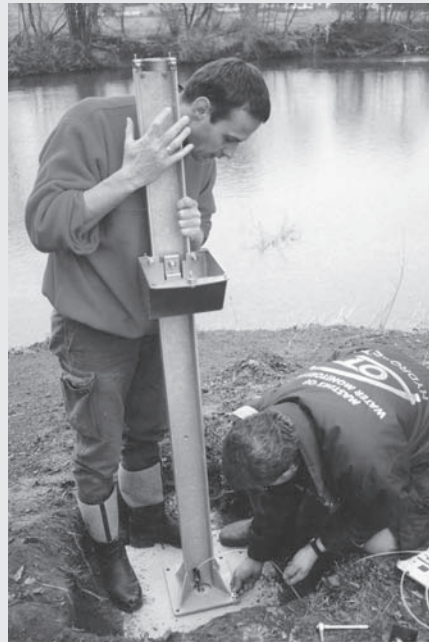
Secure stand to concrete foundation ...
