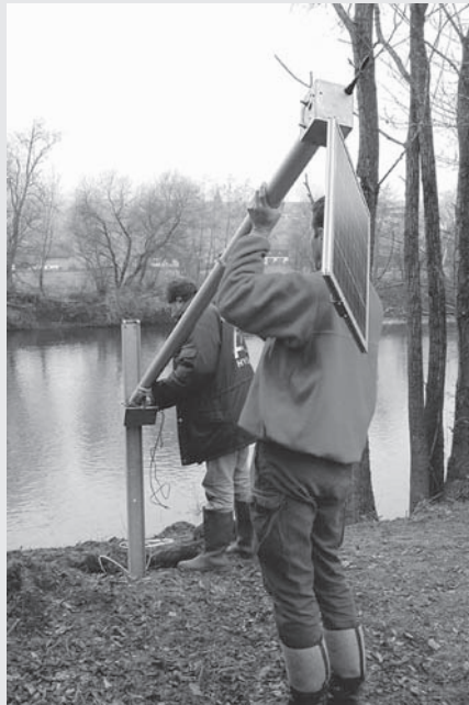
... insert pole with solar panel and GSM antennae into the stand ...
